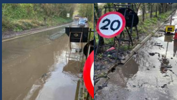
B4234 – Kerne Bridge Gully Uncovered
