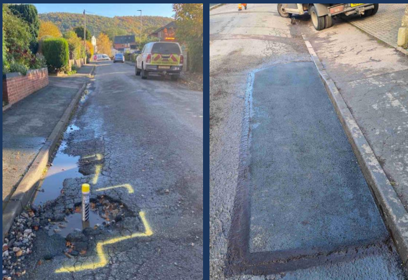
Emergency pothole repair Ryefield Road
